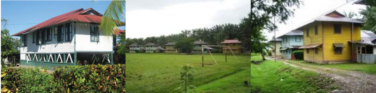
FIGURES 8-9-10. Buildings and housing complexes in Coto 47, Corredor district, 2010. (ProDUS)
