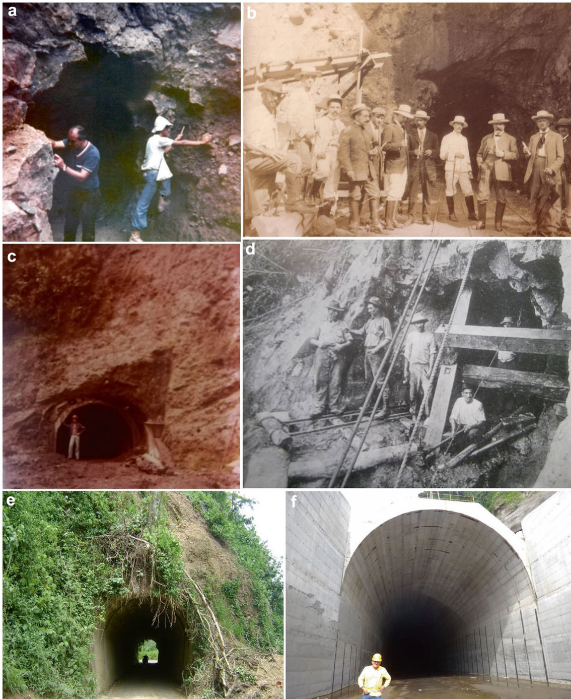
Fig. 12.9 Tunnels. a Gold tunnel at Tres Hermanos Mine in 1975, Juntas de Abangares; b the former Costa Rican president, Cleto González (third from right to left), possibly at the Cambalache tunnel along the Pacific railroad, around 1909; c Zurquí pilot tunnel in 1980 cutting volcanic breccias and two volcanic dykes (~5 m thick);
