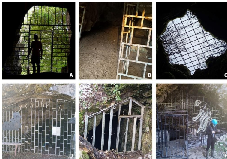
Figure 3 Improper gate design: A - the gate at the Musinska Cave allows bats to fly in and out, but it is not optimal. B - the cave at the entrance of Kalna Matnitsa Cave remains open to allow bat access. C - The Kaletto Cave entrance is equipped with a gate, that might stop bats, but does not stop visitors. D - The gate at the Uhlovitsa show Cave is still waiting for its renovation. E - Although the intention of the gate at the Bratanova Cave entrance is to protect bats, it is built without consulting with the EUROBATS recommendations. F - The gate at one of the entrances of the Magurata show cave. Photo credit: S. Deleva
