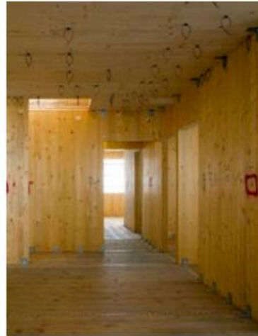
Easy fixing of services to ceiling.
