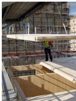
Floor panel installation.
