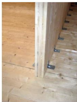
Wall panel anchored to floor panel.
