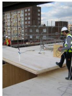
Floor panel installation.
