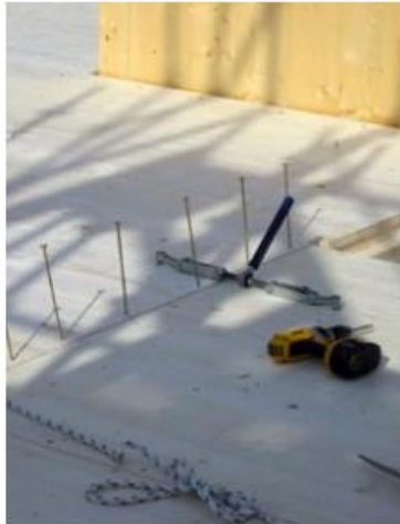
Self-drill woodscrews installed using lightweight power drivers.
