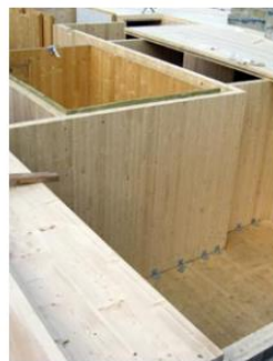
Typical internal wall arrangement.
